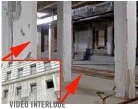
Tour Downtown's Huge Hall of Justice Rehab, Underway Now
